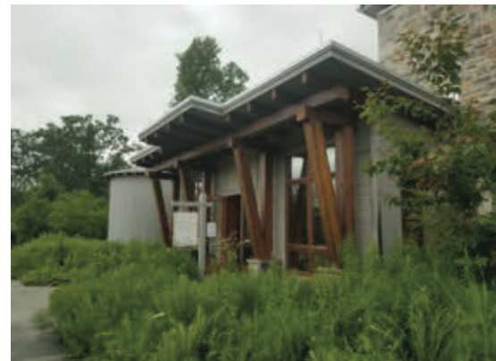
LEED Platinum, Living Building Challenge Certified, Gladstone NJ - Host site of East Coast Green 2019
